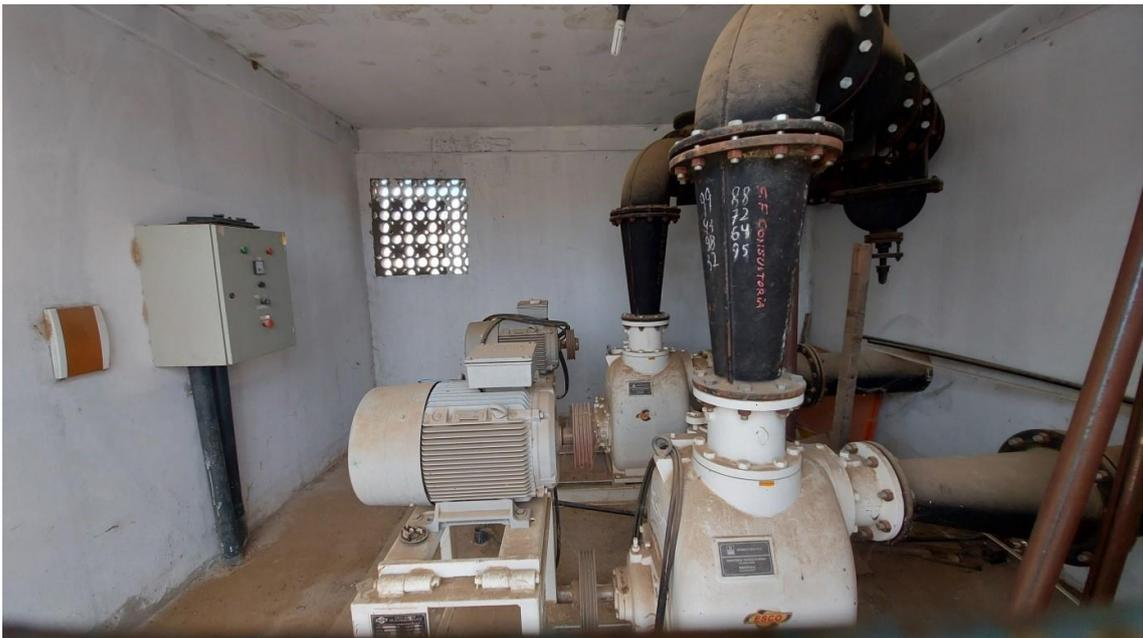
**Figura 28 – ETE Abandonada, Bombas de Recalque**
